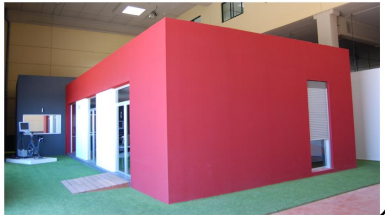
Figure 5 - Indoor and outdoor views of the CIAMI Living Lab
