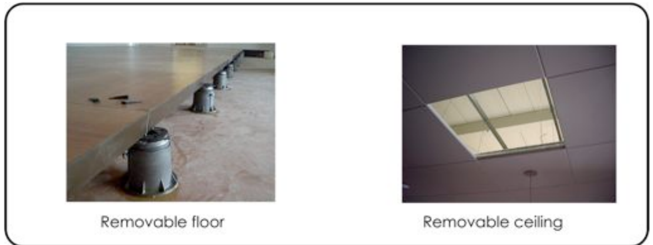
Figure 4 - Removable floor and ceiling modules at CIAMl Living Lab
